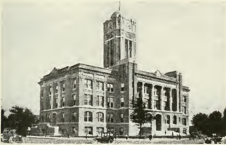
JOHNSON COUNTY COURT HOUSE, CLEBURNE
