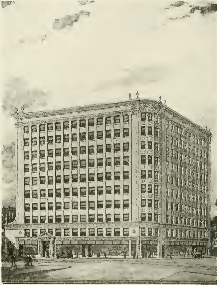
N. P. ANDERSON & COMPANY BUILDING, FORT WORTH
