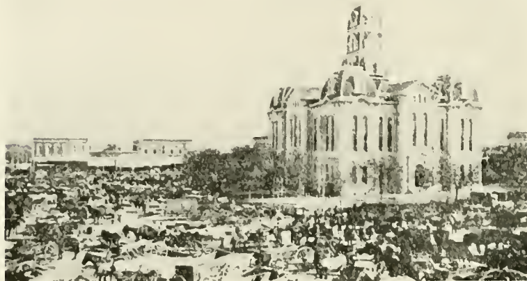
COURT HOUSE, WEATHERFORD
